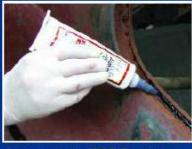
Squeeze a bead of **POR PATCH™** into seam.
