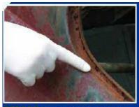
BEFORE: Rusted, leaking seam.
